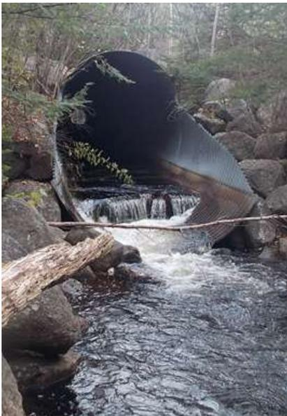
*An example of a site where remediation is planned for this summer. This culvert will be retrofitted with an additional baffle and a chute into the plunge pool. Button Brook, Annapolis Co.*
